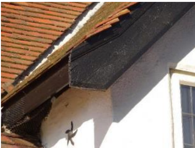
28 – Timber soffit and fascia board
