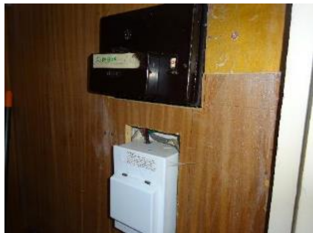
57 – Electrical fuse board
