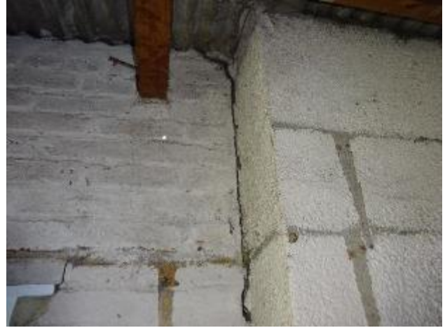
72 - Settlement/ movement cracking
