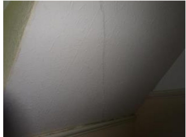
33 - Thermal cracking to plaster
