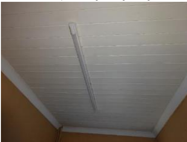
37 - Timber ship lap finish to utility room
