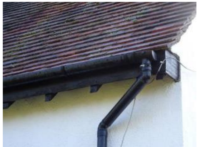
29 – Timber soffit and fascia board
