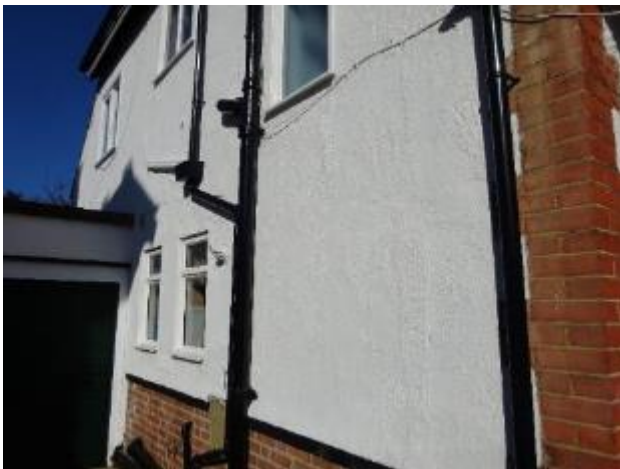
15 – Rendered finish to side elevation
