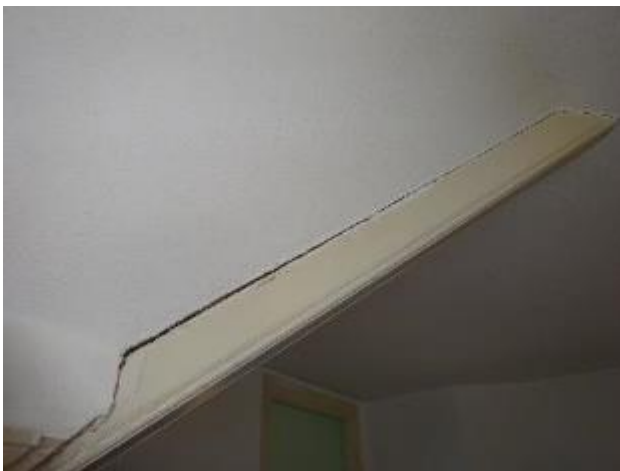
34 - Thermal movement adjacent to front valley
