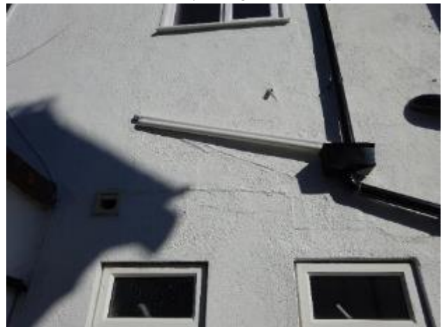
16 – Localised hairline cracking to side elevation
