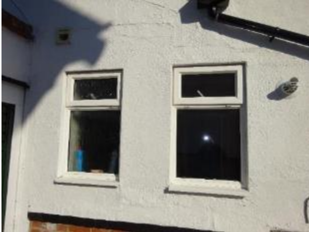
25 - uPVC windows to side elevation
