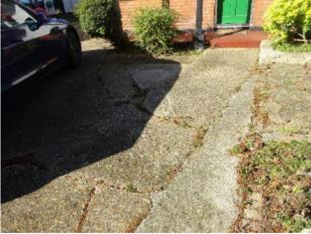
62 – Heavy cracked hardstanding concrete
