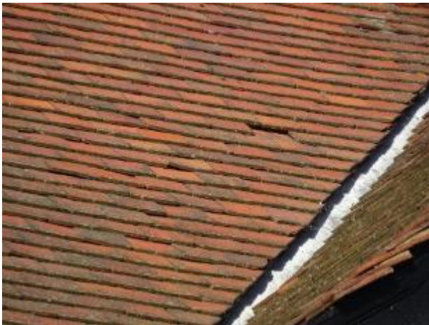
5 – Slipped/ damaged tiles to front
