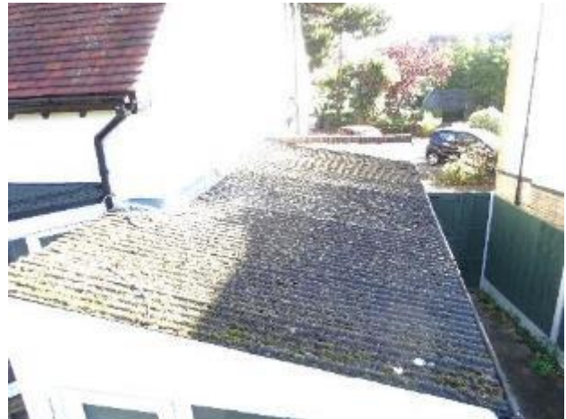
68 - Asbestos profiled roof
