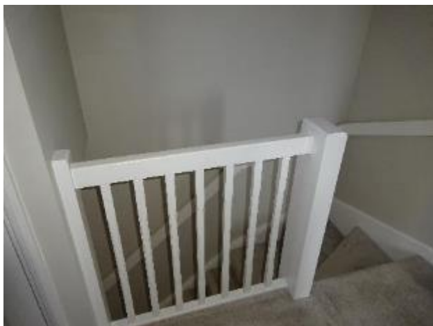
38 – Timber balustrade to landing
