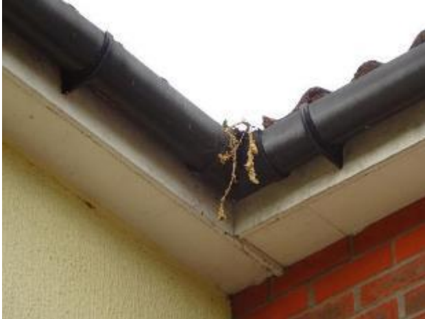
5 - Vegetation growth within gutter to front
