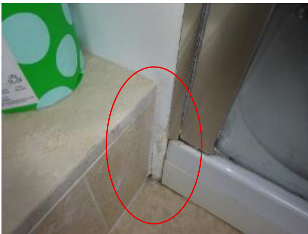
47 - Water damage
