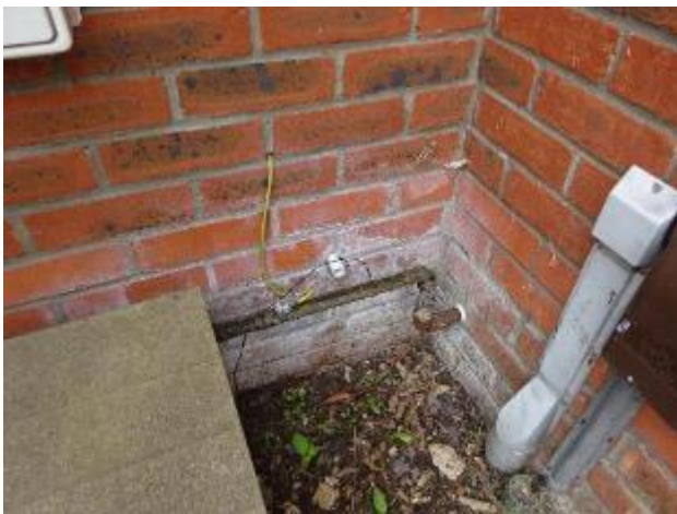
9 - Staining to brickwork
