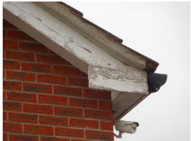
20 – Timber soffit and fascia board
