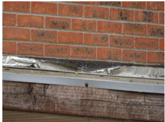
56 - Loose flashing
