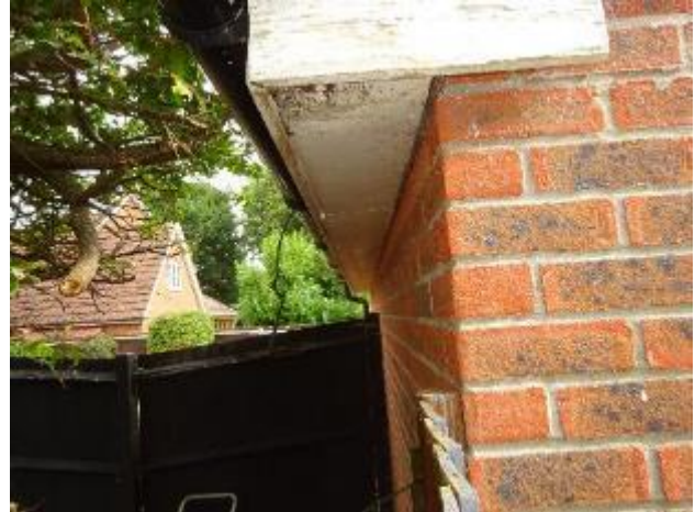
58 - Timber soffits and fascia board
